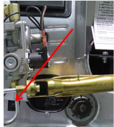
*If the water heater does not work, make sure the power switch (indicated by the red arrow, located by removing the exterior water heater door) was not inadvertently switched OFF.*
