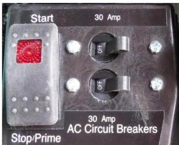
*The output from the generator may be interrupted if the main generator circuit breakers trip. These breakers are located on the main generator control panel (remove the cover on the generator to access). If there is no power when the generator is running, check and reset these breakers.*
