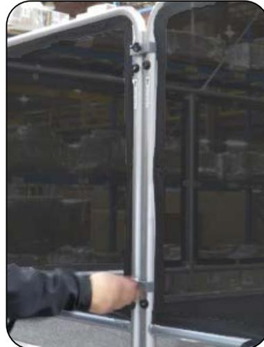
7. Then screw in the top and bottom locks *as shown*, to secure the end gates in the closed (locked) position.
