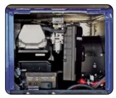
Generator with Front Panel Removed to Access Main Power & Circuit Breaker.
