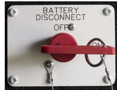
*Typical battery disconnect switch*
