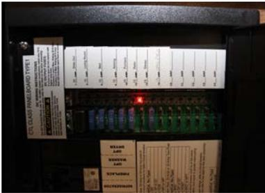
*A red light (as shown in the above photo), typically indicates a blown or missing fuse in the load center.*
