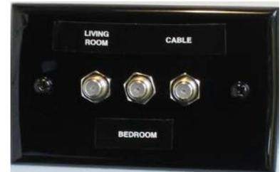
*Typical exterior cable and satellite connection plate, located in the utility center.*
