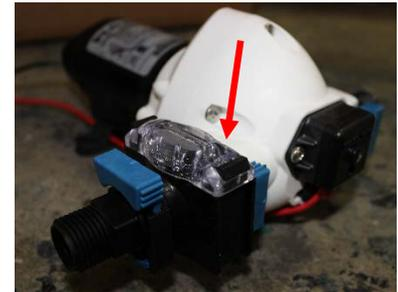
*Periodically unscrew and remove the access cover behind the utility center to access the water pump filter (indicated by arrow). The water pump filter has a removable, reusable screen that needs to be cleaned of dirt and debris as routine RV maintenance.*
