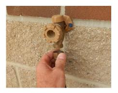
Disconnect garden hose from "TANK FLUSH" inlet.
