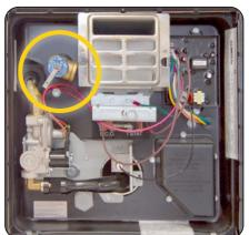
Inside the Exterior Door Dometic Water Heater
