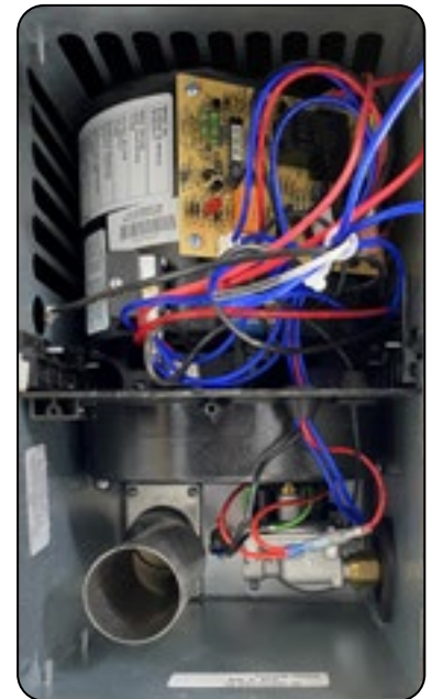
Furnace w/Outside Panel Removed
