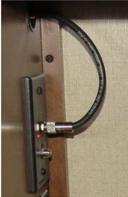
*Typical TV signal booster, located in the cabinet to the right of the living room TV in the Solitude 369RL. In the photo, the ON/OFF button is to the right of the coax cable.*
