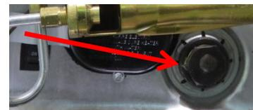
Typical anode rod, installed
