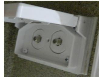
*Typical cable/satellite outlet. The satellite coax connection is located on the left and the cable coax connection is located on the right.*
